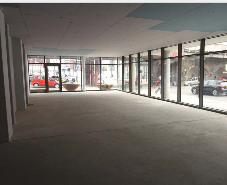
Internal view of the unit currently in shell and core condition
